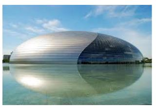
About the building one can on the internet read: It is a curved building, with a total surface area of 149,500 square meters, that emerges like an island at the center of a lake. The titanium shell is in the shape of a super ellipsoid with a maximum span of 213 meters, a minimum span of 144 meters and a height of 46 meters). [1]
